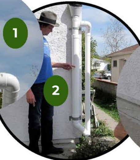
First Flush Diverter
