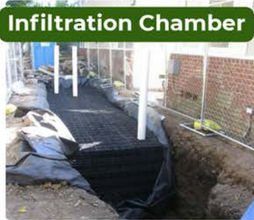
Infiltration Chamber
