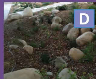
Slight depression, berms, and boulders of a typical swale
