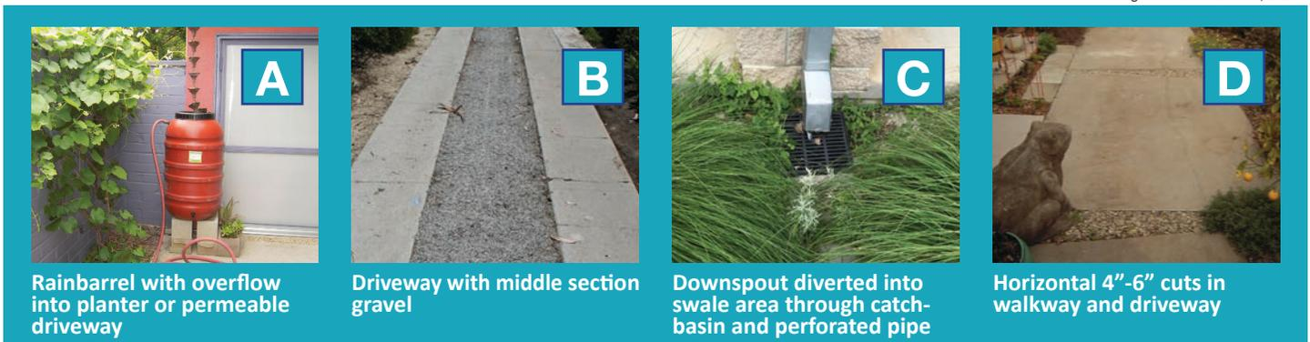
**A** Rainbarrel with overflow into planter or permeable driveway
