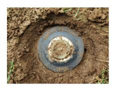
2. For each sprinkler head, you want to measure the distance between that head and its adjacent heads.
