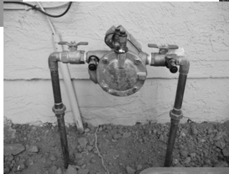
Reduced Pressure Vacuum Breaker
