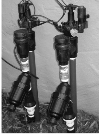
Anti-siphon valves - drip
