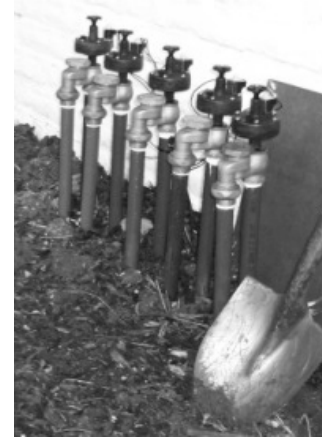
Anti-siphon valves - spray
